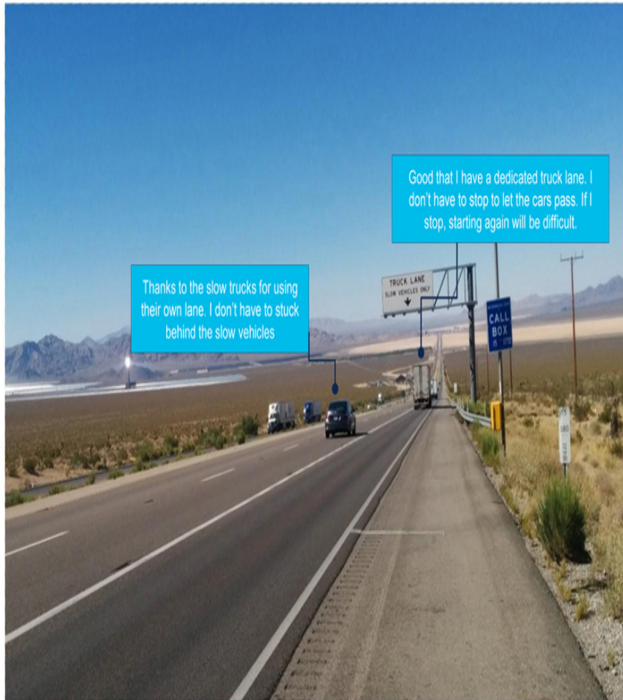
Figure 6-5 Traffic and congestion segregation to dedicated lanes.
